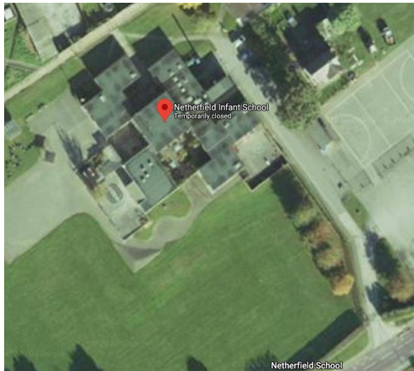
An aerial view of school
